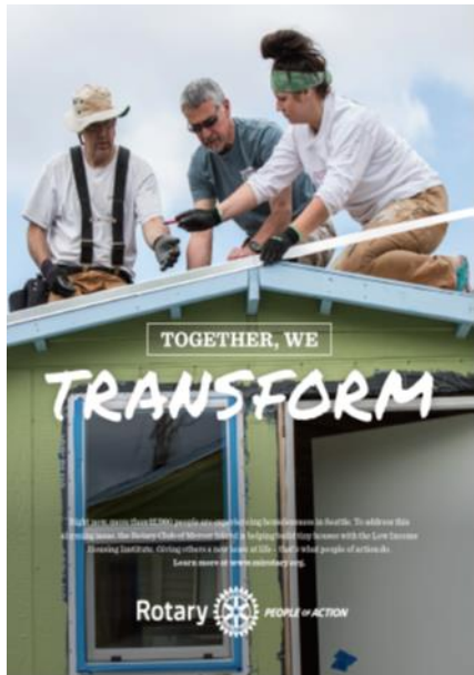
Rotary members work together to build the roof of one of the tiny houses donated by the Rotary Club of Mercer Island.
